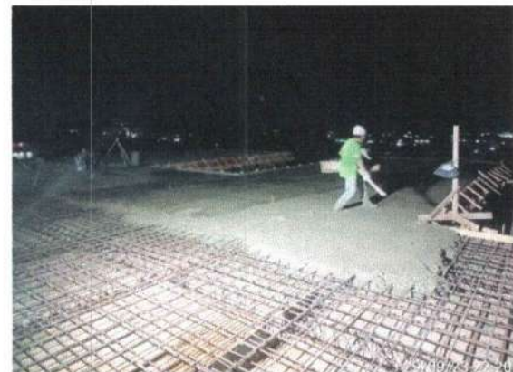
Pengecoran Drop Panel
