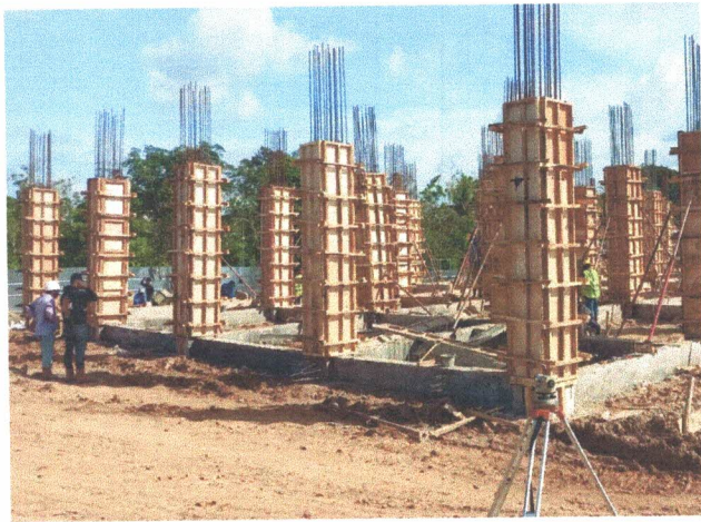
Bekisting Kolom K6 60 x 60
