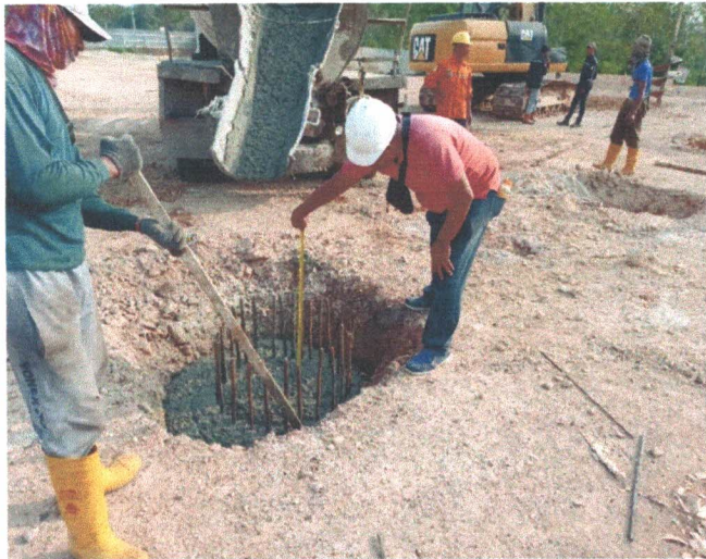
Pengecoran Bore Pile
