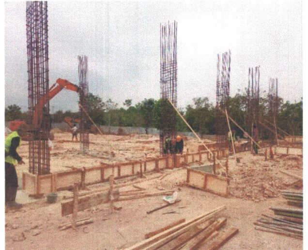
Bekisting Tie Beam
