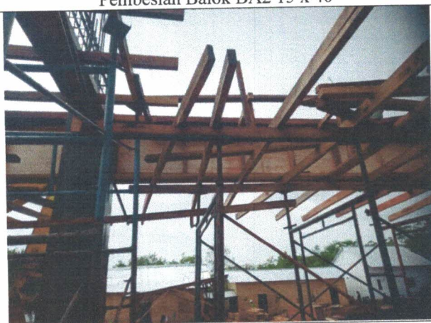
Bekisting Balok B1
