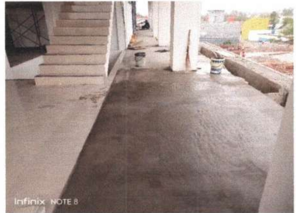
Pekerjaan Water Proofing Lantai 2
